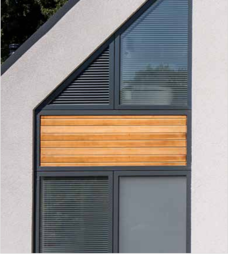
VELFAC 200 FAÇADE WITH LOUVRE PANEL AND NON-VENTILATED CEDAR PANEL
