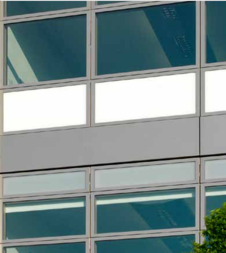
VELFAC 200 FAÇADE WITH LOUVRE PANEL AND NON-VENTILATED CEDAR PANEL
