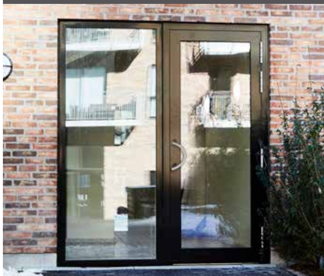
2-LEAF ESCAPE DOOR WITH PANIC BARS AND CLOSERS IN A VELFAC 200 SCREEN
