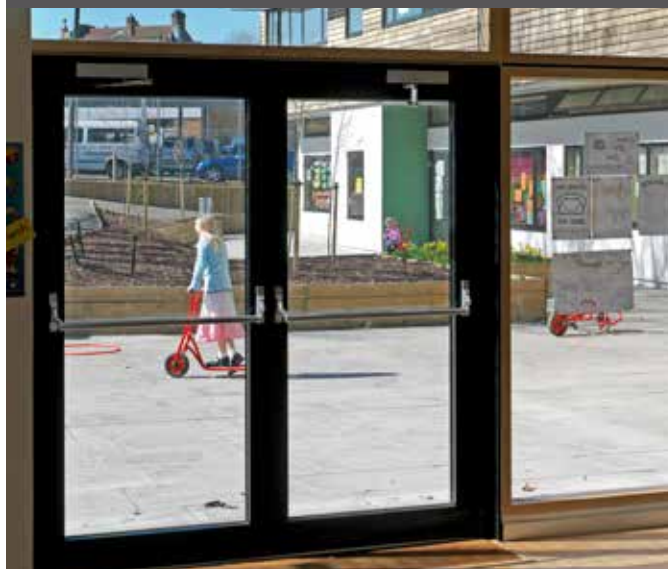
2-LEAF ESCAPE DOOR WITH PANIC BARS AND CLOSERS IN A VELFAC 200 SCREEN
